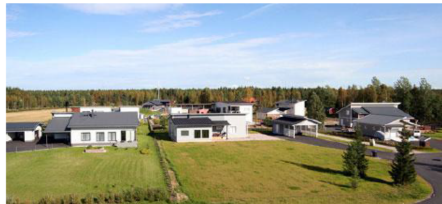
CHP Plants Alpuja, Finland Volter 30
