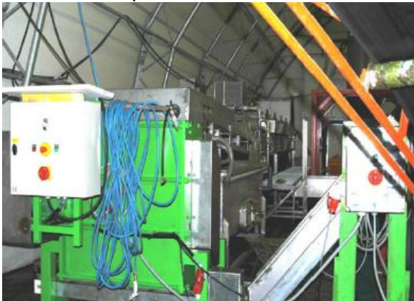
Florafuel AG plant
